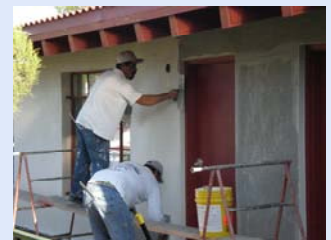
In the picture above the workers are placing the foam insulation on the wall. The picture below, the workers are putting the final color coat of stucco on the wall.
